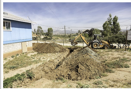
septic work has begun
